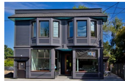
Glasswood Commercial TI is the first Commercial Passive House Retrofit in the United States
